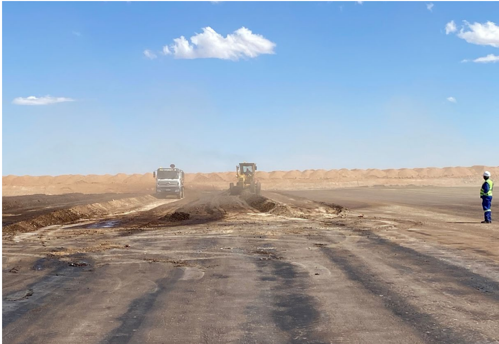
Dust control project at customer site
